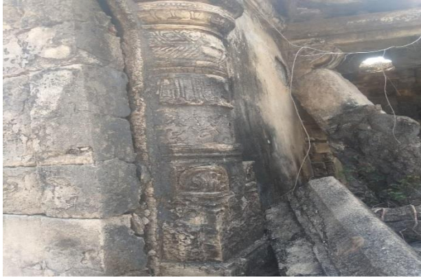
Inner Pillar in a dilapidated condition
