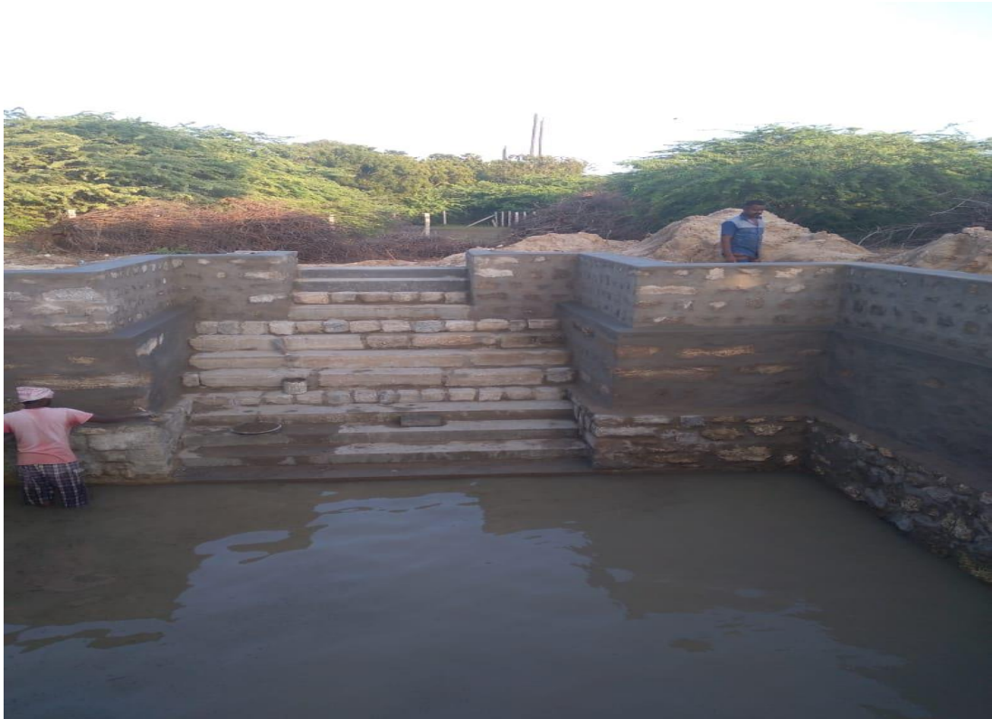
Strengthening the base, pointing work and the parapet wall
