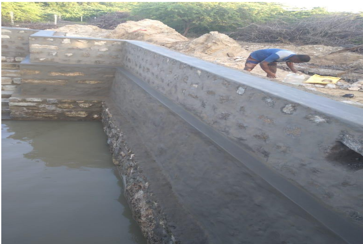
Strengthening the base, pointing work and the parapet wall
