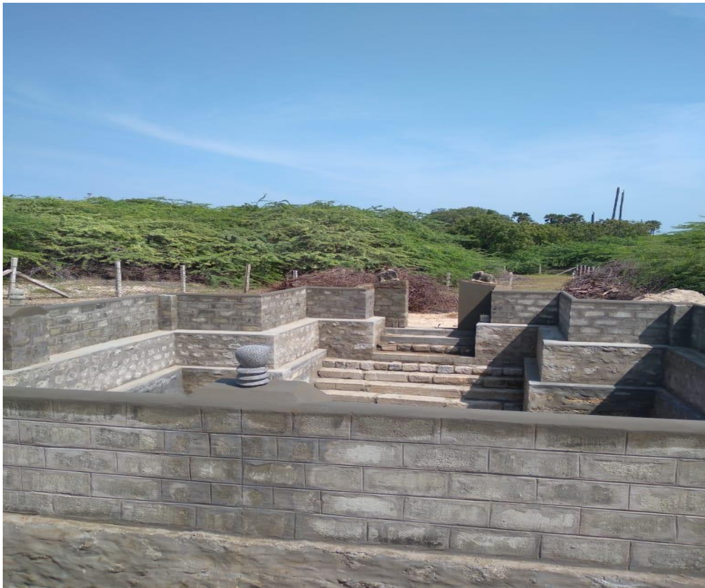
More height of the parapet wall to avoid sand and soil entering the water body
