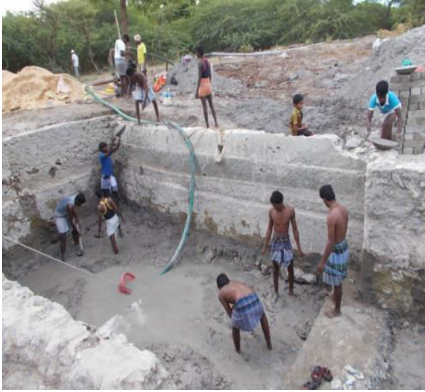
Jnanavapi Teertham - Removing the water and cleaning the sludge and construction of side wall
