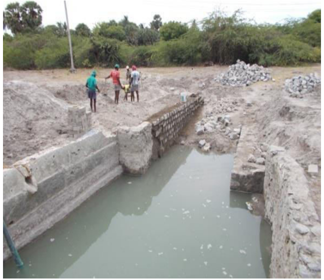
Jnanavapi Teertham - Removing the water and cleaning the sludge and construction of side wall
