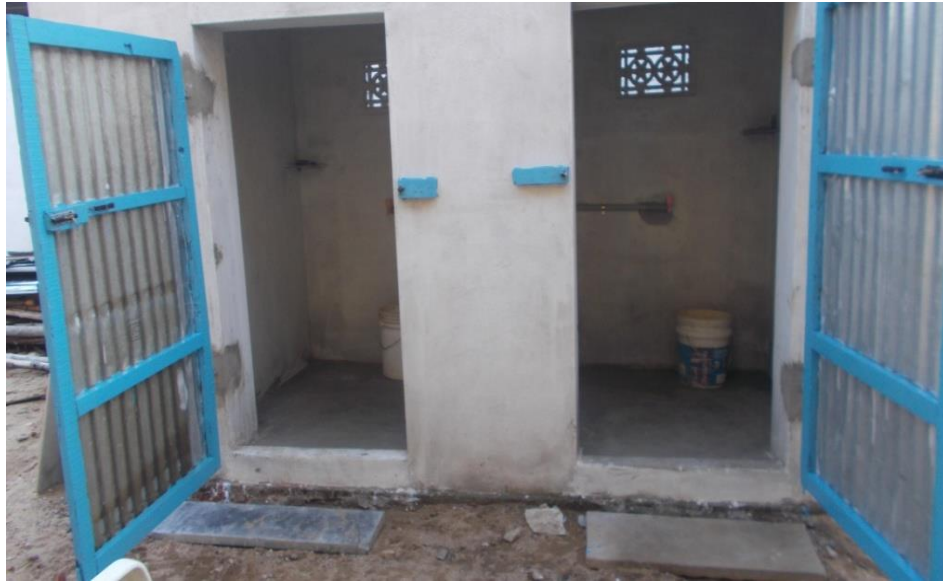
Two bath rooms at the back side of the building
