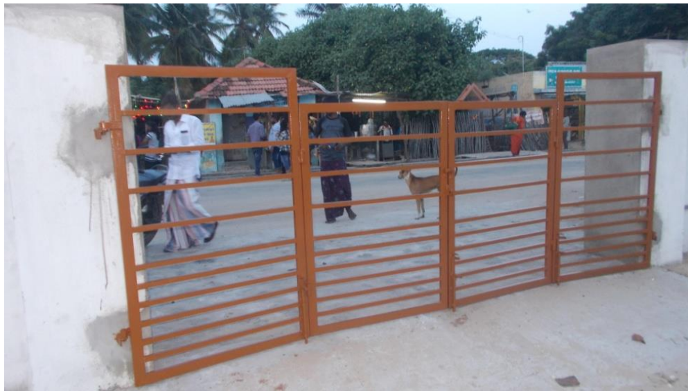
Strengthening and colouring of the main gate
