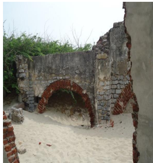
Fig.5: Destroyed post office
